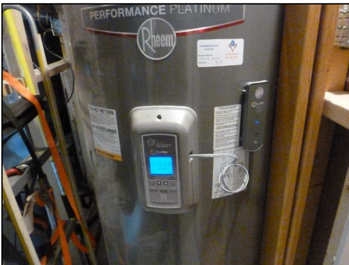
67. Tank water heater
