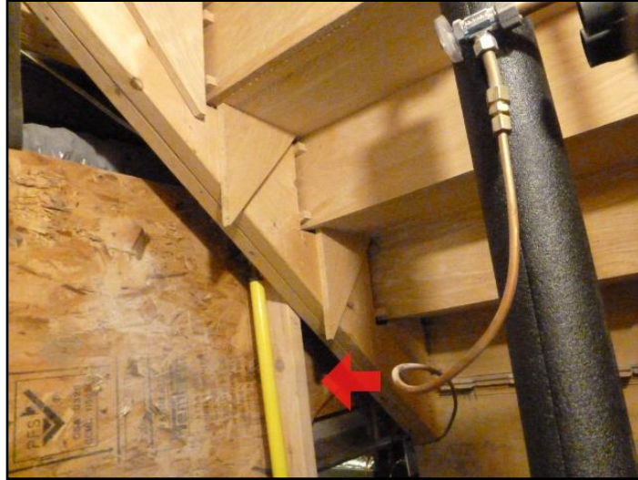
45. insufficient support
