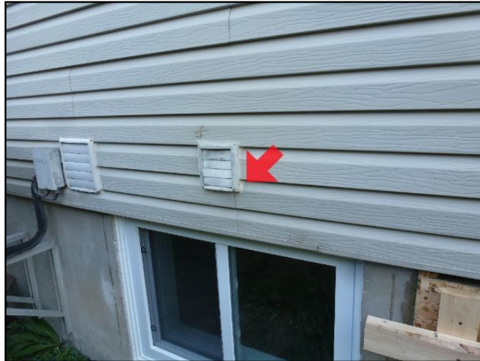
21. Deteriorated caulking
