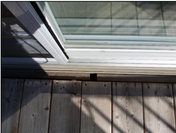
28. Missing ledger board
