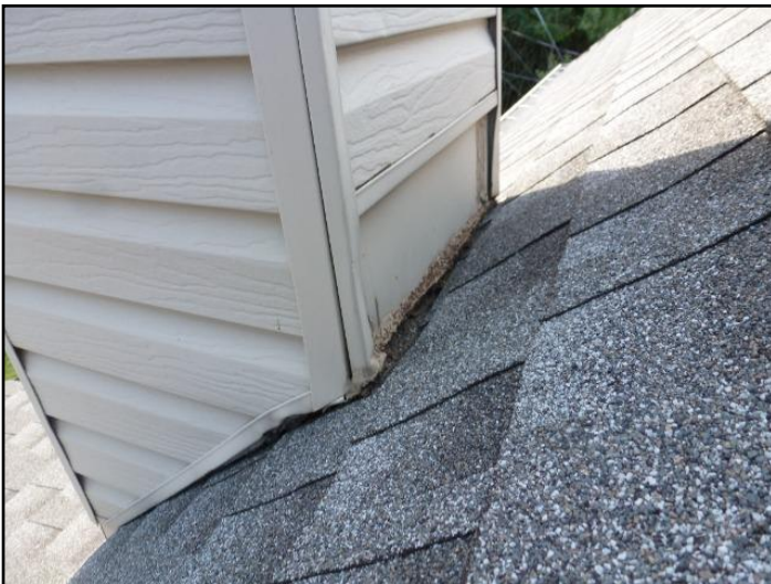
6. Improperly sealed
