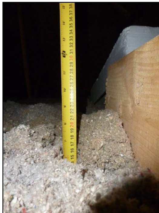
64. Cellulose insulation
