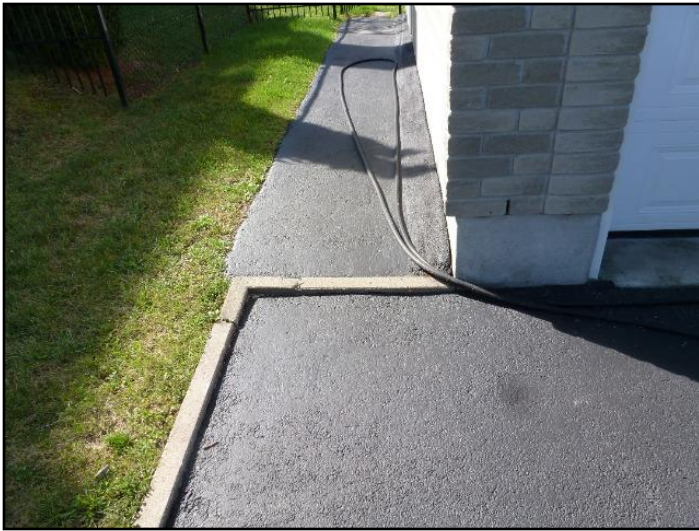
35. Improper slope or drainage
