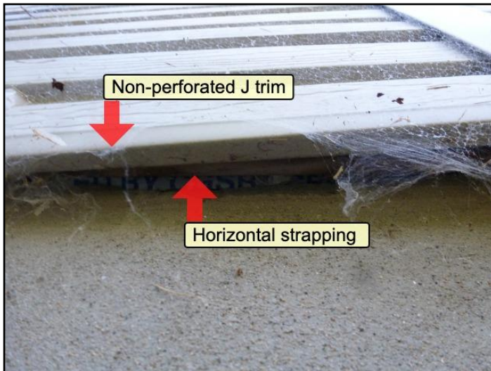
18. Improperly install siding
