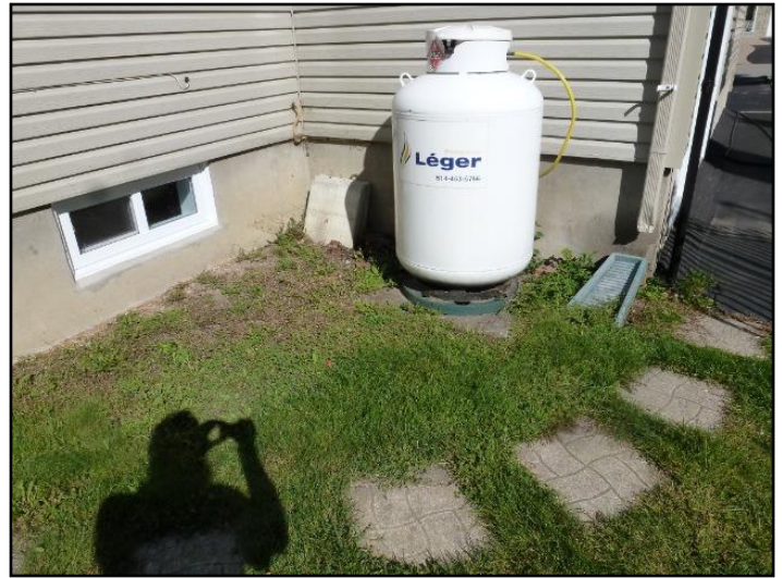
36. Improper slope or drainage
