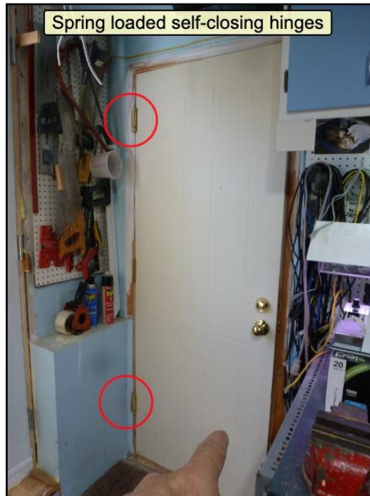
82. Fire door doesn't shut
