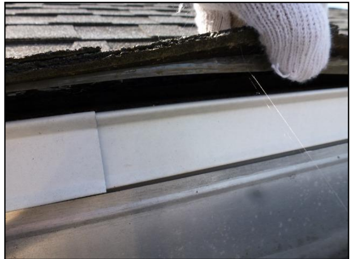
3. Improperly secured drip edge
