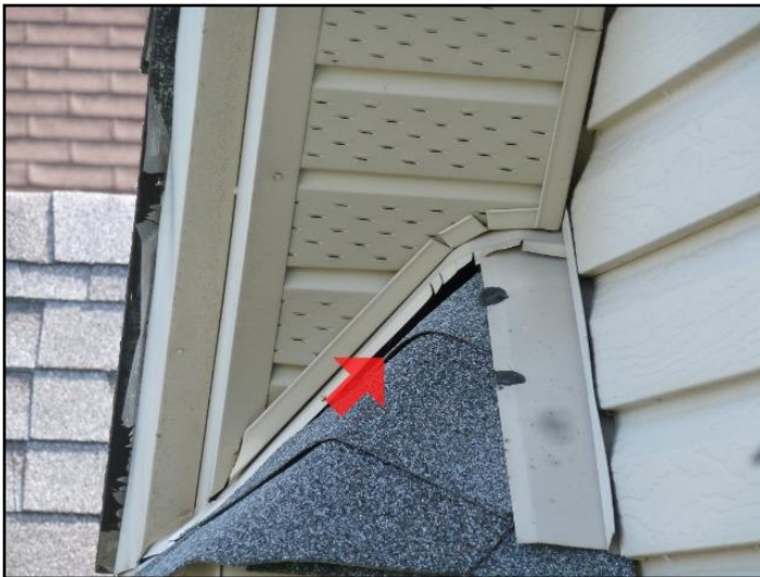
2. Flashing too far from roof surface
