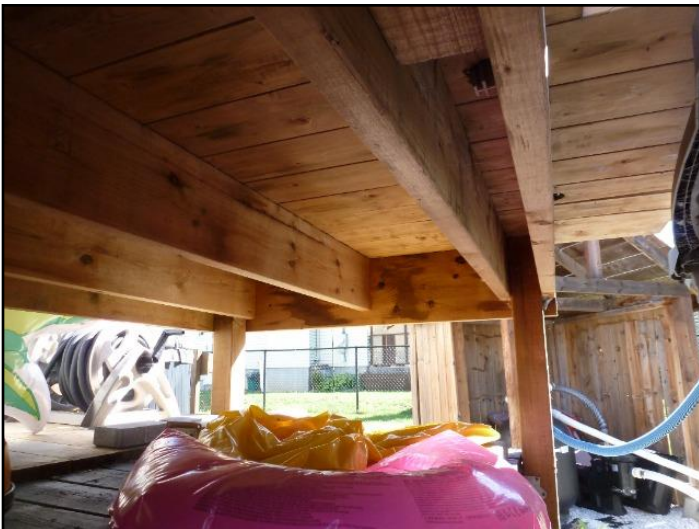
32. Missing joist hangers
