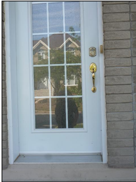
22. Paint and Caulking - deteriorated / missing
