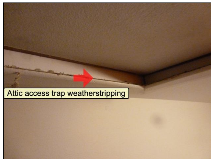
65. Damaged seal
