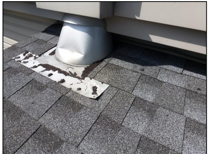
7. improperly installed chimney flashing
