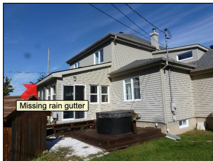
13. Missing rain gutter
